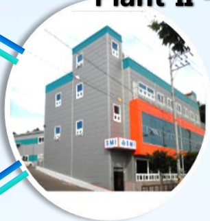
Plant III – Pup Joint Factory Chilgok-gun, Korea
